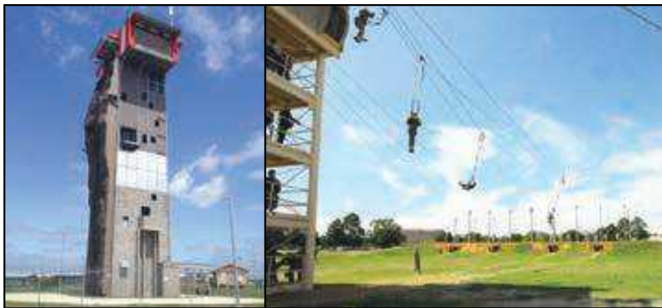
Figure 6: Mock Tower Training
